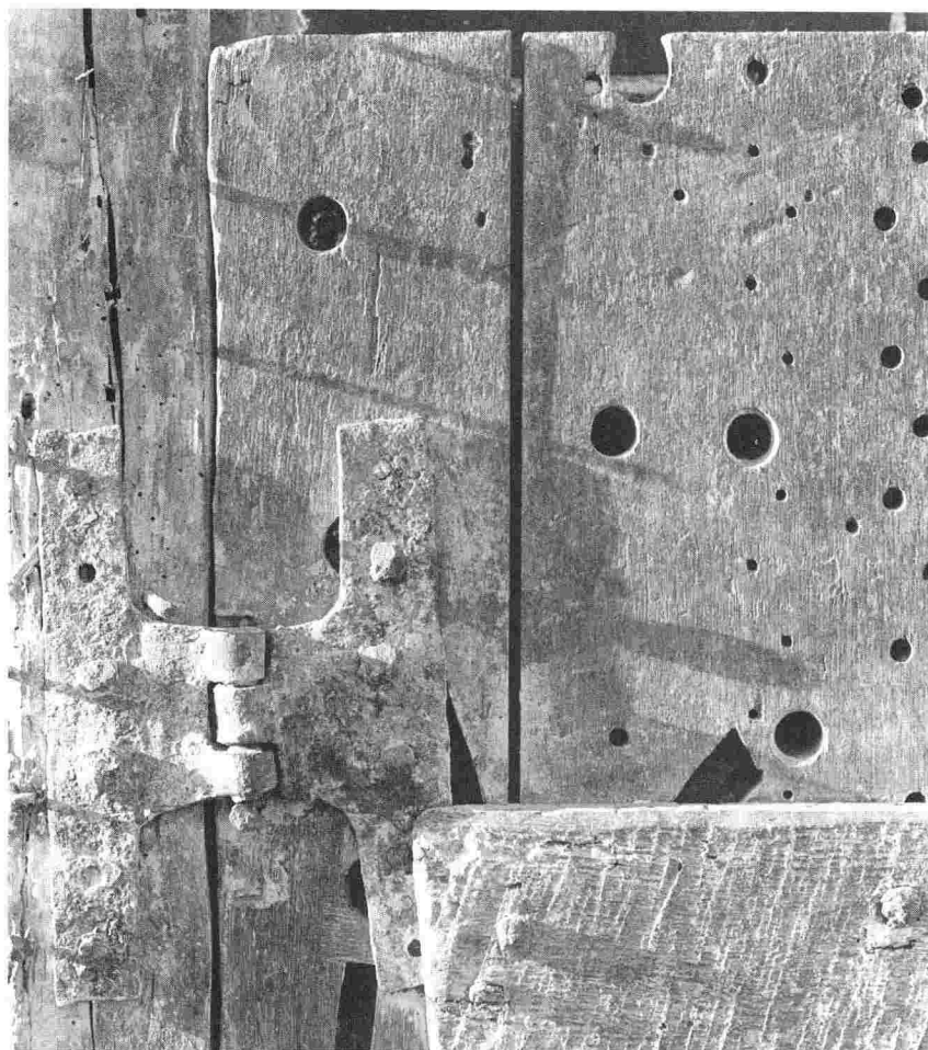
PLATE XXVI – Detail of top corner at the back of the door, showing 17th-century hinge under part of door ledge.
