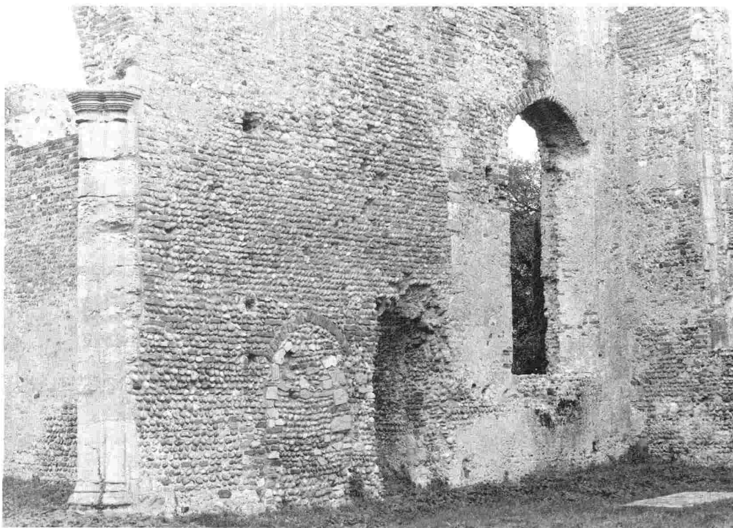
PLATE XXXII – Looking towards the north side of the chancel, Walberswick. The blocked door to the vestry can be seen next to a later opening. The vertical line of sockets nearest to the nave can be seen to the left of, and above, the door arch.
